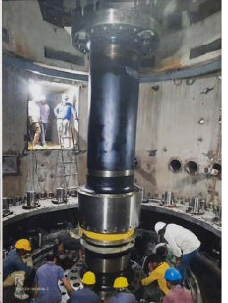
Yedula Pumping Station Pump House-Erection of Unit
