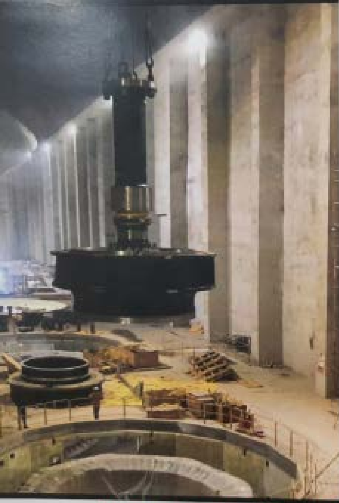
Yedula Pumping Station Pump House-Erection of Unit
