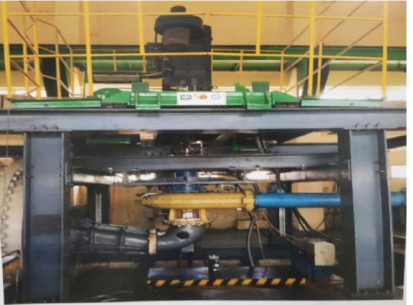
Yedula Pumping Station Pump House- Model Testing at BHEL, Bhopal
